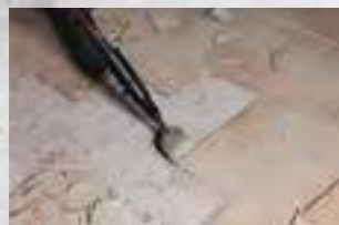
Ceramic Tile Removal
