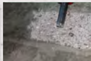
Roughening Concrete
