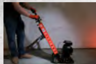
Coating & Corrosion Removal
