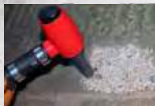
Reducing Levels on Concrete
