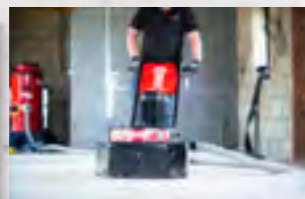
Removing High Spots
