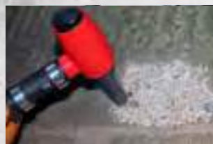
Reducing Levels on Concrete
