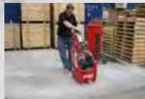
Reducing Levels on Concrete
