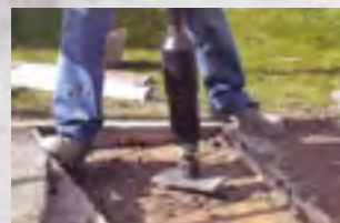
Back Fill Compaction
