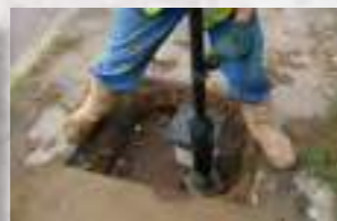
Reinstatement Compaction
